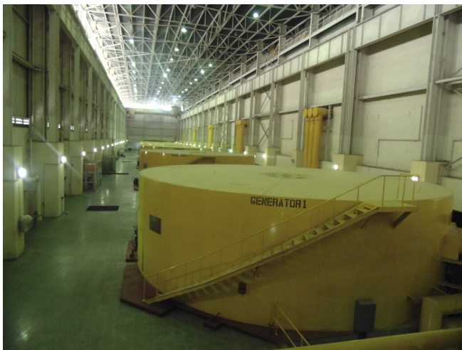
One of the generators
